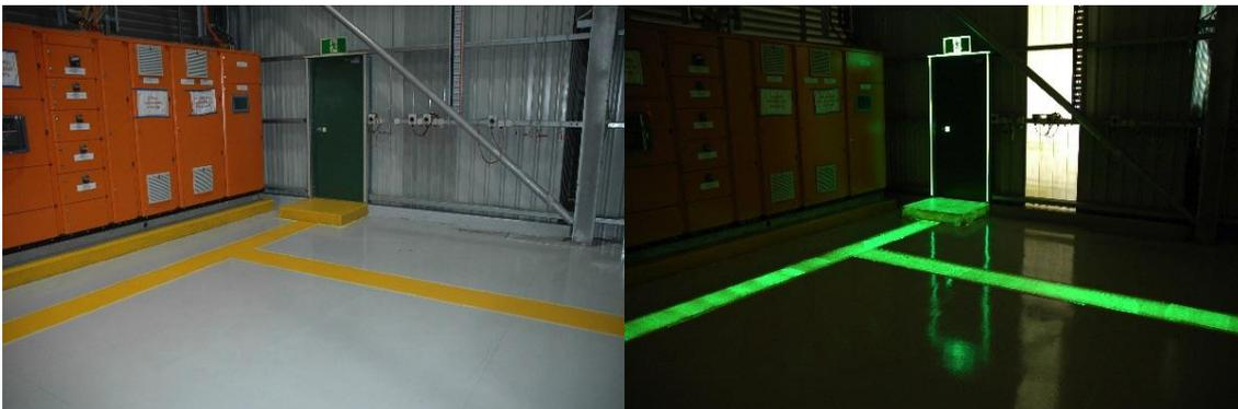
Figure 2: A PL Exit sign and other PL technology at a VISY site in NSW
