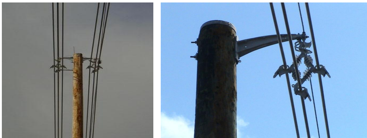
Figure 23: Covered wire with support wire
