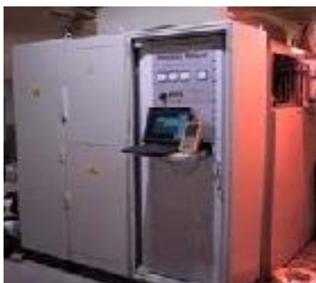
Figure 13: Example of a REFCL
