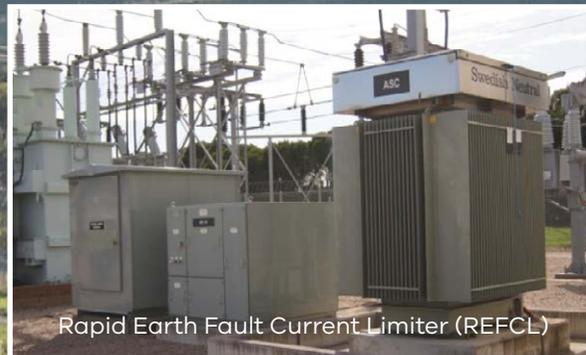
Rapid Earth Fault Current Limiter (REFCL)
