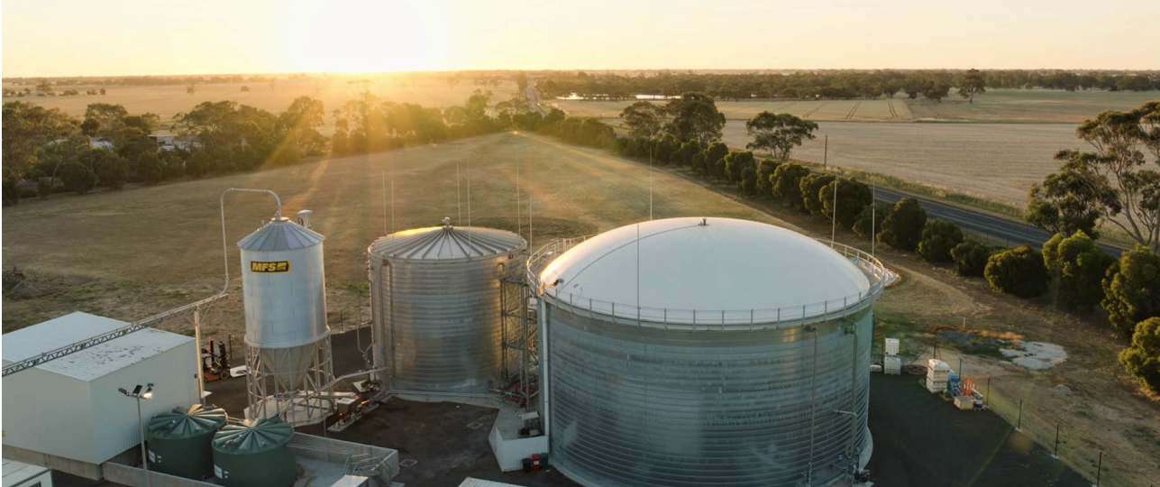
Blue Lake Milling Bioenergy Plant – Bordertown, South Australia (image source: Delorean Energy)
