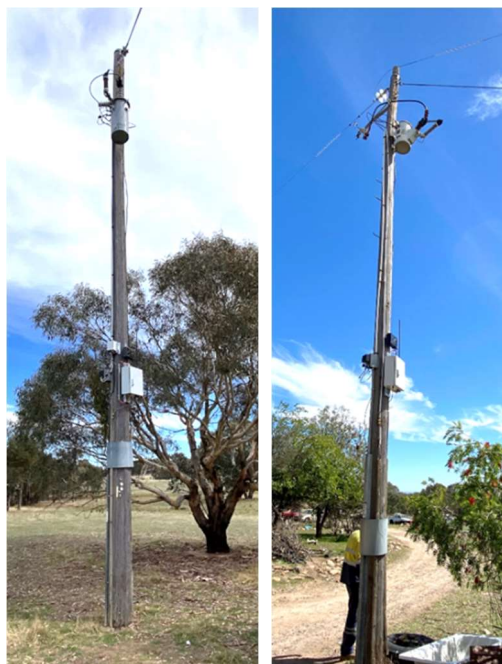
Figure 6: Modified Generation 3B EFD units (NB: no high-voltage sensor) installed on SWER customer substation poles
