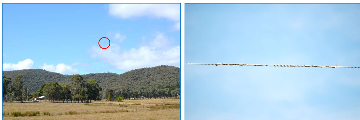
Figure 21: Defective splice on Wodonga Blacks Flat SWER Path C-D
