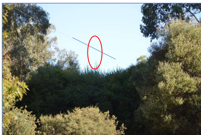
Figure 19: Vegetation close to Wodonga Cencic SWER powerline on Path A-B
